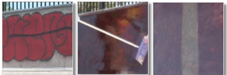
Feltpen Fadeout removes red spraycan stains from virtually any building surfaces, after or during removal using BBSM Graffiti Remover.
