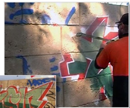
After applying the Coating, it is easy to remove graffiti with hot water alone, or with just one quick application of our removers.
