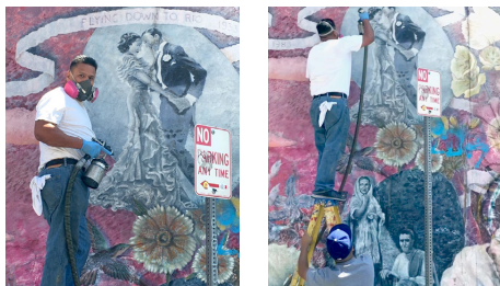
MURALSHIELD being applied with HVLP sprayer
