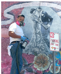
MURALSHIELD being applied with HVLP sprayer
