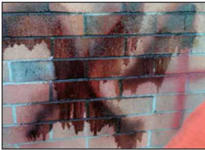
Red spray paint dissolving with BBSM
