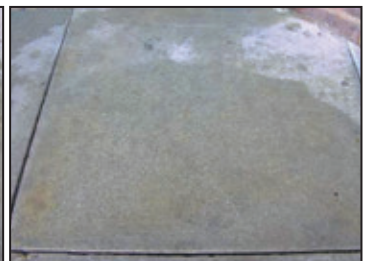
Then brush on Feltpen Fadeout and leave on while the remaining stain fades away. Rinse away once complete
