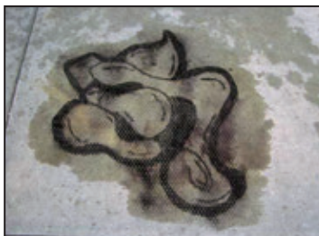
First, dissolve what you can using Bare Brick, Stone and Masonry Graffiti Remover
