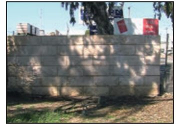
Graffiti is removed using just hot water at 2000psi / 2-3gal per minute
