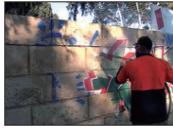
Graffiti is removed using just hot water at 2000psi / 2-3gal per minute
