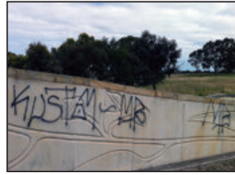
Decorative Sound Walls
