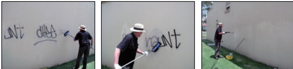
On a damp wall, brush on BBSM then rinse away
