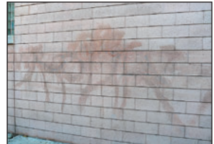
This 'anti-graffiti' coating actually made removal even more difficult in the long-term
