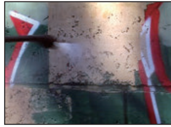
Graffiti is removed using just hot water at 2000psi / 2-3gal per minute
