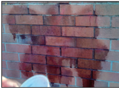
One application of FPFO
