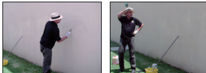
Touch up any remaining areas of undissolved graffiti using SSGR
