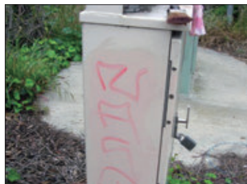
Brush on Feltpen Fadeout to fade away remaining ink stain
