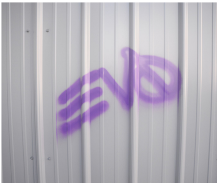
BEFORE: Spray paint graffiti markings on surface coated with Valspar ASTM-compliant coating.
