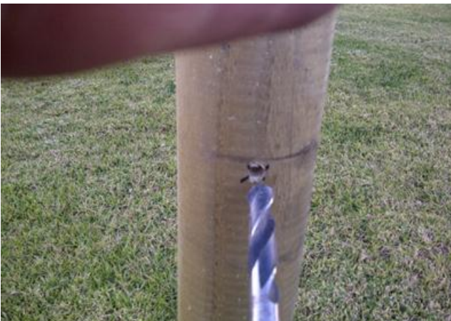
Upsize hole with 16mm drill bit 50mm deep
