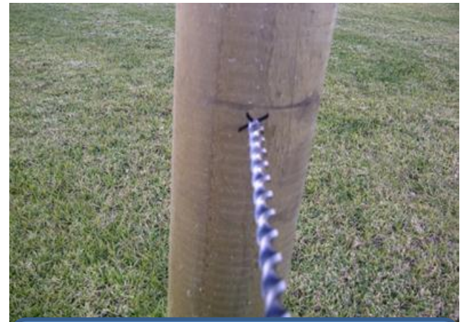
Using 8mm-10mm bit drill through post
