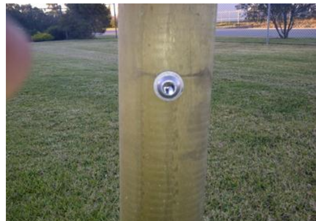
post is ready to accept anchor
