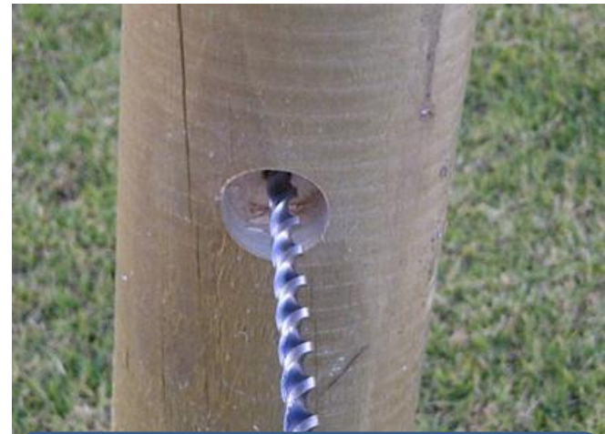
Using centre mark, drill through the post 8mm-10mm
