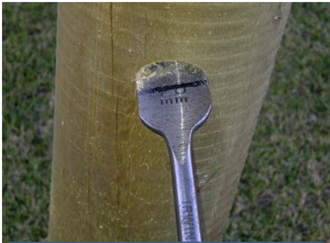
Drill to pre-marked depth to take anchor
