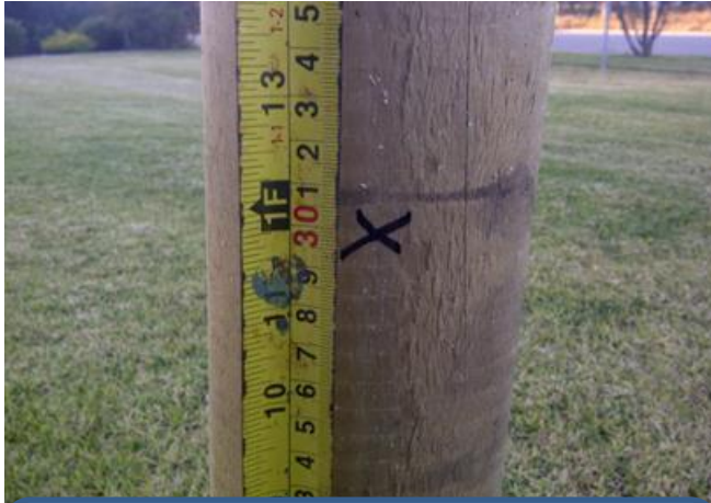
Mark Fence strand spacing
