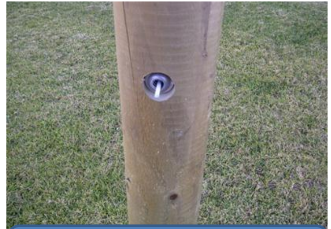
Anchor installed, recessed into strainer post
