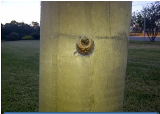
The strainer post is now ready to take the anchor
