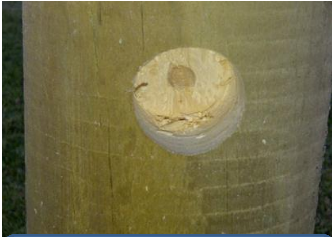
Rebated and 10mm hole ready for upsizing
