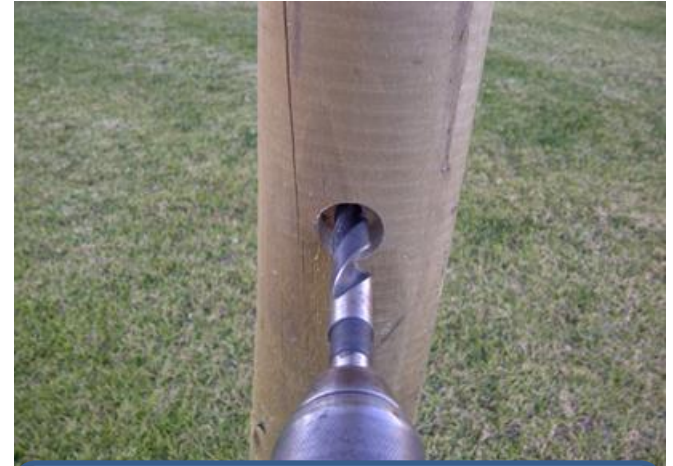
Using 16mm bit upsize hole to a depth of 50mm
