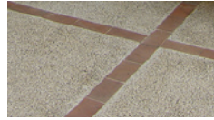
Decorative cement & bricks
