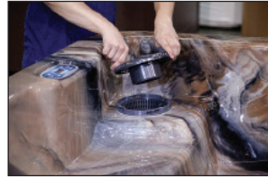
Remove housing ring.
