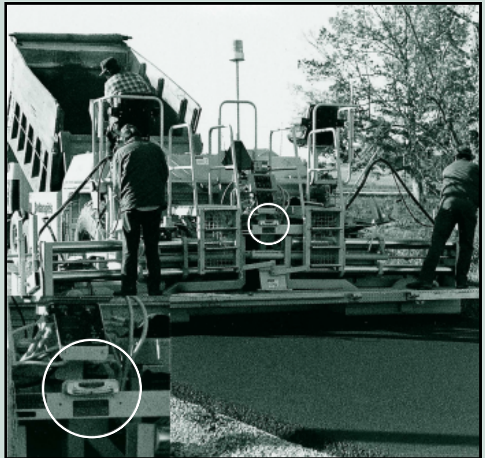
Paving (Photo courtesy of Cedarapids, Inc.)
