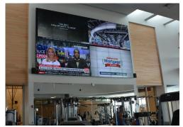
The solution presented was an impressively large 7x7 28.5-foot video wall, consisting of 49 Barco 55" LCD displays seamlessly aligned and hung using Peerless-AV's DS-VW755S Full Service Thin Video Wall Mount with Quick Release
