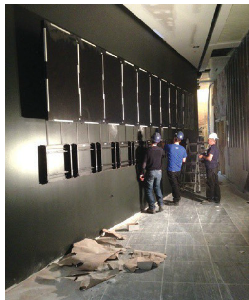
To seamlessly install multiple video displays, Cablage Expert relied on the tool-less adjustability of the Peerless-AV mounts—a top feature for the team.
