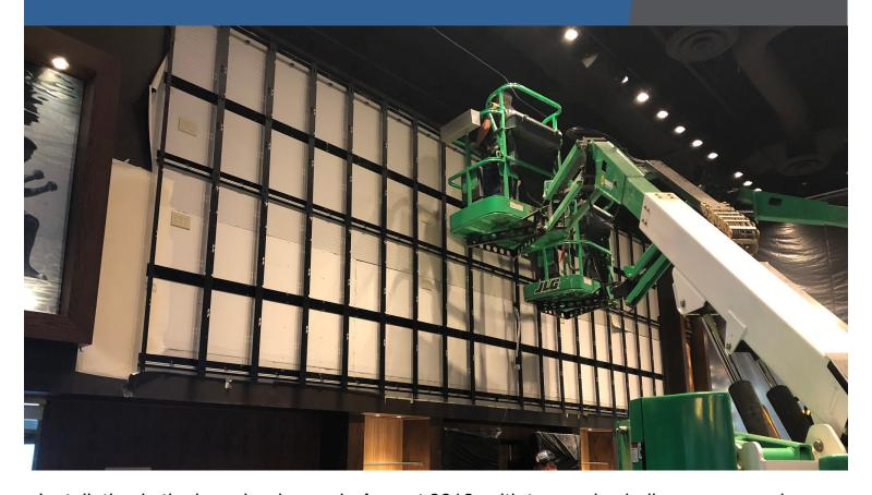
Installation in the busy bar began in August 2018, with two main challenges: a very heavy display and an uneven wall. With a display weighing almost 1,500 pounds and a crooked wall, engineers were required to complete back bracing, which involved tearing into the sheet rock to install support kickers to the studs. Once the wall was deemed safe to handle the weight of the giant TV and mount, the wall was then patched and installation commenced.
