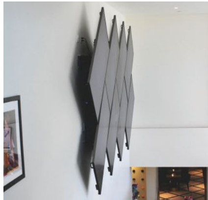
Integrator Fluid Sound used Peerless-AV's Special Purpose Video Wall Mount for the custom video wall above the TCL Chinese Theatre's lobby escalator, and a Wall Kiosk Enclosure for displays outside each cinema, in tandem with NEC 75- and 43-inch sets.
