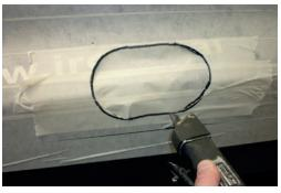
7. Drill mounting holes to 16mm.
