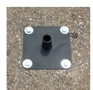
Tighten hex screw until head securely holds base plate in place
