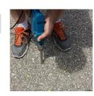
Use high speed power drill with 3/4" masonry bit and core drill each hole 6" in depth.
