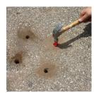
Using the wide flat hammer stuff mungo plugs into core drilled holes.
