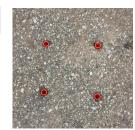
Make sure top of mungo plug is flush with asphalt surface.
