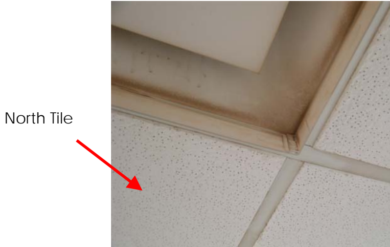
Figure 16: North tile with deflector after 201.7g of dispersed ball clay powder
