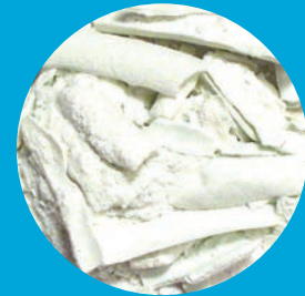
CALCIUM AND MAGNESIUM LIMESCALE DEPOSITS
