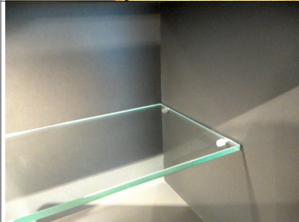
Shelf support covered with plastic to prevent scratching of the glass.
