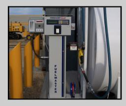
The system is composed of a Central Controller PC, a fuel management unit (as seen in photo below), and a secure access device such as a smart card, credit card, or a programmable key. Depending on what information your organiza-tion needs to track, FuelMaster will provide custom reports to suit your needs.
