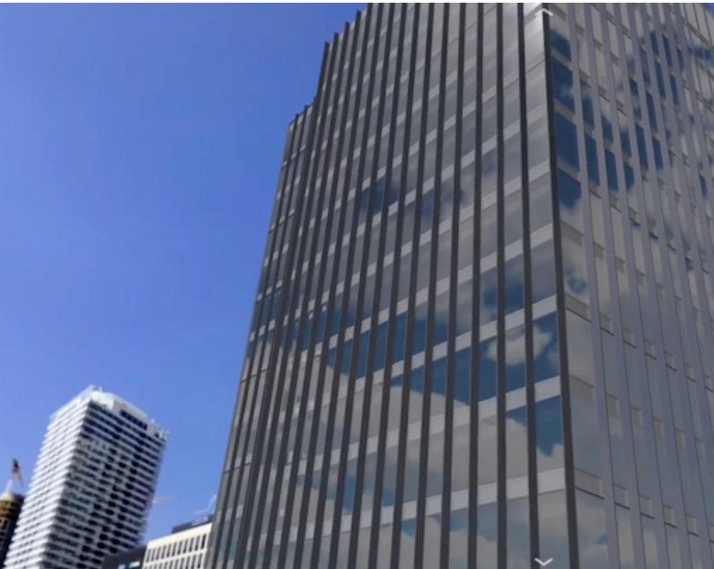
Boston Properties visualize fins of varying depths, reducing costs by $220K
