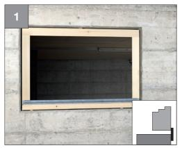
Window installed flush with the outside surface
