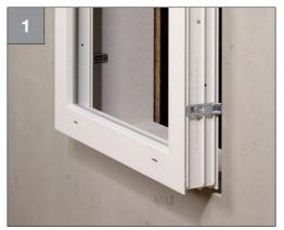
Window installed on the outside surface
