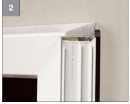
Suggestion: Mount a wedge for better water discharge ≥5°. Observe the manufacturer's specification
