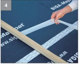
• Separate the backing strip and press the counter batten down
