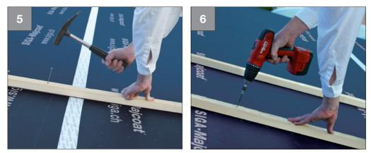
• Finally mount the roof underlay membrane by screwing or nailing the counter battens to a solid support
