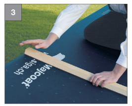
• Align the counter batten with the backing strip folded back on the roof underlay membrane
