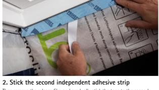
Then remove the release film and gradually stick the tape to the second surface (in this case, onto the window reveal).
