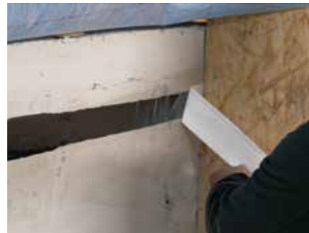
2. Remove backing paper to expose adhesive
