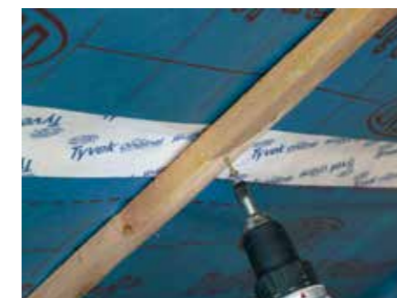
14. Press batten into position and permanently fix
