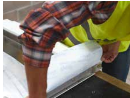
2. Fold the exposed tape strip back and apply to the frame
