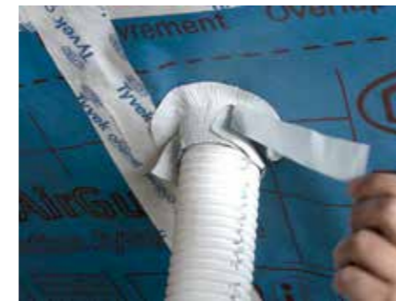
7. Once wrapped around, remove remaining release strip
