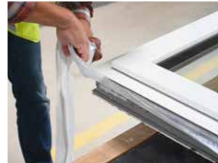
3. Form a loop on the corners: 1.5 x joint width. Seal or press together firmly
