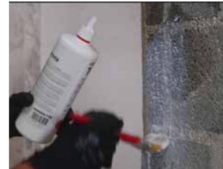
1. If the wall surfaces are chalky and need to be stabilised, apply Tyvek® primer
