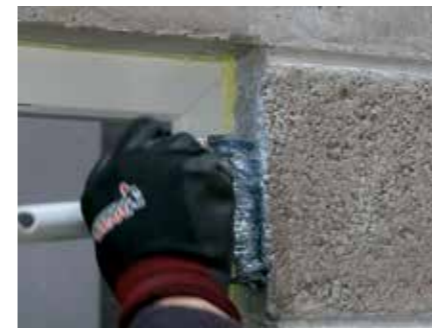
7. The primer is white on application, but will turn transparent when it cures after 1 hour approx.
