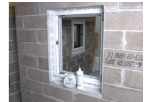
13. Repeat the process for the internal side of the frame and the gap is sealed!
