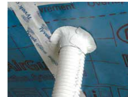
8. Make sure Tyvek® FlexWrap EZ is bonded to both the pipe & the AVCL
