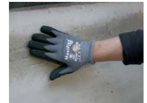
6. After an hour the primer turns transparent
