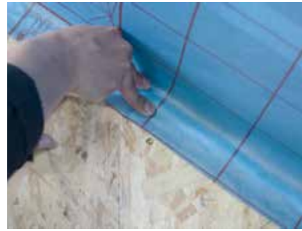
2. Lap the membrane onto the sealant and apply pressure with fingers either side of the bead. Ensure that the sealant is not pressed flat as a bead thickness of at least 1mm should be maintained
