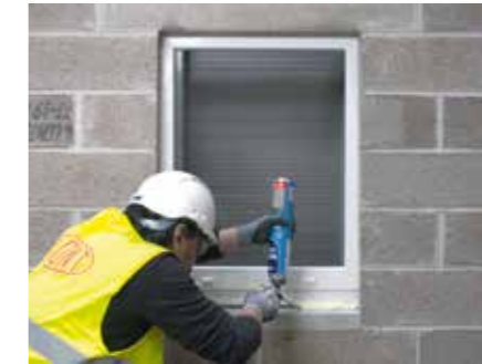
2. Shake can thoroughly and apply DuPont™ Insta Stik™ into the gaps around the window
