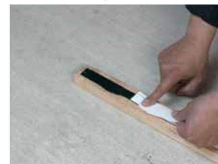
13. Remove release liner
