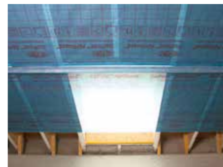
9. Extend AVCL over any windows or doors (to be trimmed later)
