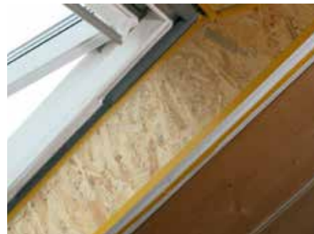
4. Tape should also be applied tight up to window/door frames
