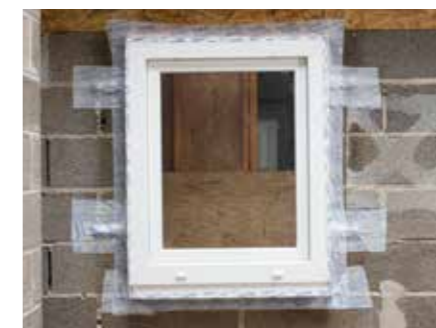
11. Tape over any exposed brackets and the sealing work is complete
