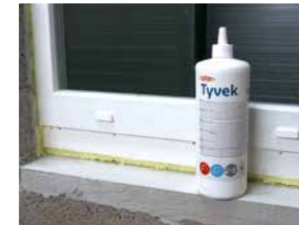
5. If the surfaces around the frame need to be stabilized Tyvek® Primer can be applied to improve adhesion for sealing tape
