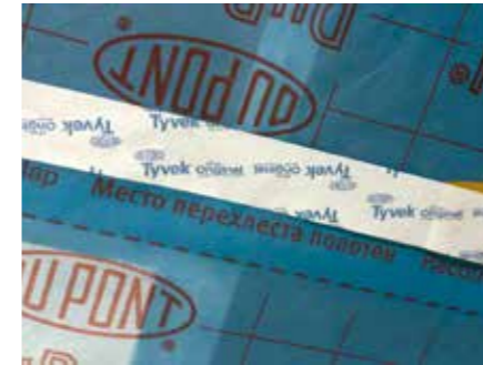
10. Seal laps with Tyvek® Tape (Tyvek® Metallised Tape should be used with DuPont™ AirGuard® Reflective or AirGuard® FR System Tape should be used with DuPont™ AirGuard® A2 FR fire retardant AVCL)
