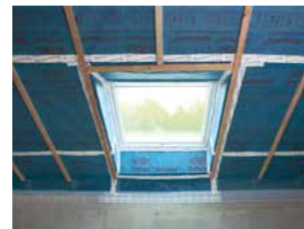
19. All sealing work can be easily checked by a visual inspection
