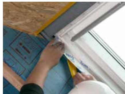
8. Bond tape to frame and remove remaining release paper
