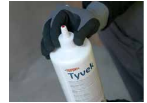
3. Use Tyvek® Primer to stabilise the surface and improve adhesion for the adhesive tape
