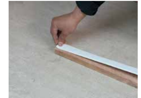
12. Apply Tyvek® Butyl tape to batten
