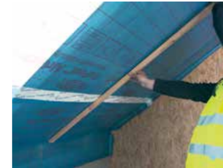
11. Measure battens prior to fixing
