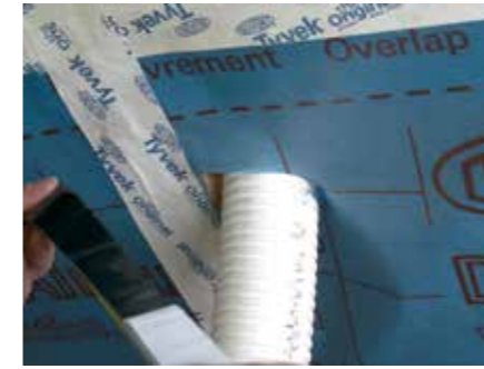
1. Cut a length of Tyvek® FlexWrap EZ, fold in half and remove one release liner strip
