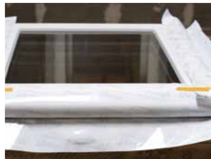
8. Fold the skirt and temporarily fix back with tape before installing the window
