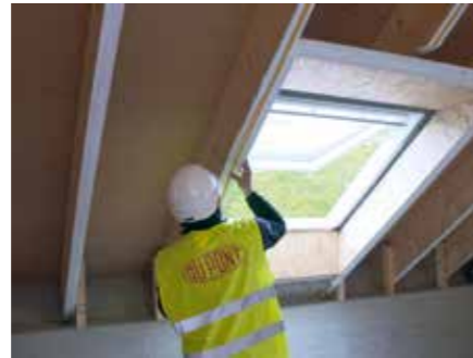
2. Apply tape to all facing surfaces . . .
