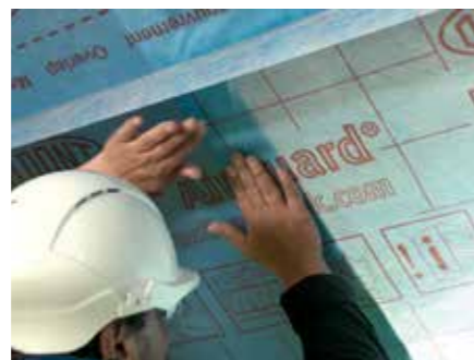
8. AVCL should be pressed firmly against tape
