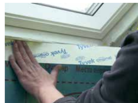
12. Seal tightly around window
