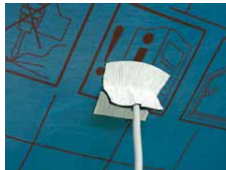
7. Remove the remaining backing strips and press together
