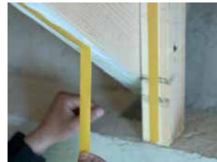
6. Remove tape release liner from the Tyvek® Double-sided Tape on all surfaces
