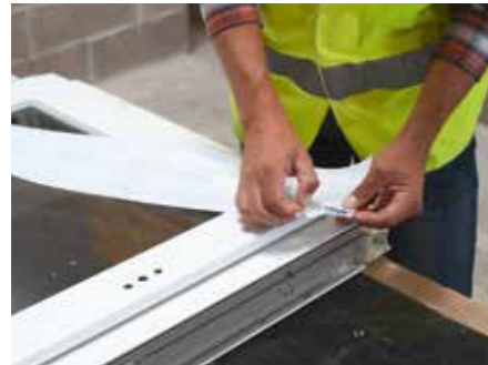
1. Using the 150mm Tyvek® Window Tape, start by removing the narrow release liner (20mm)
