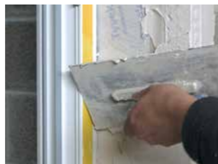
11. Tyvek® Window Tape provides a suitable key for the application of plaster or render
