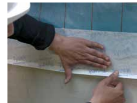
11. Cover equally the AVCL and the wall surface, removing each release liner in turn
