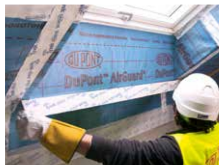
11. All cuts, laps & junctions in the membrane should be sealed with DuPont™ Tyvek® Acrylic Tape
