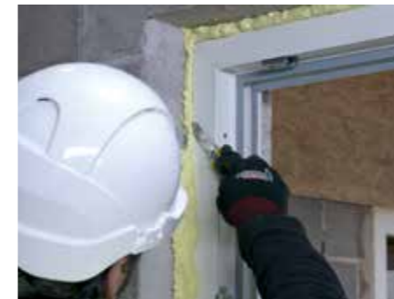
4. The spray foam will cure in around an hour and any excess can be trimmed off
