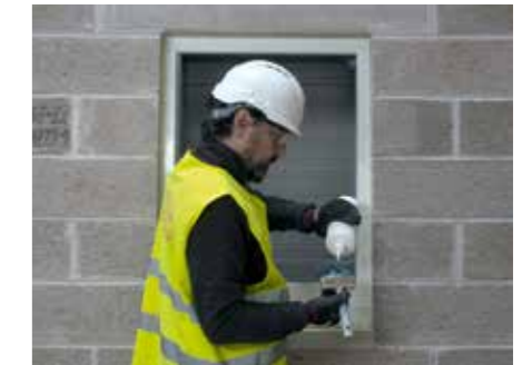
6. Tyvek® Primer can be applied onto the wall surface or directly onto the brush
