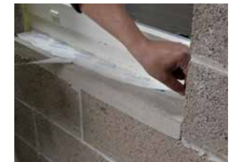
9. Starting at the cill, apply the exposed tape to the frame and remove the remaining backing strip
