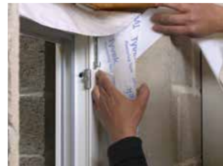
9. When the window unit is fixed into the opening remove the remaining release paper and apply Tyvek® Window tape on the interior side of the window. Finish as per page 36.
