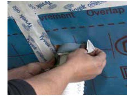
2. Wrap Tyvek® FlexWrap EZ around the pipe base, bonding the exposed adhesive to the pipe
