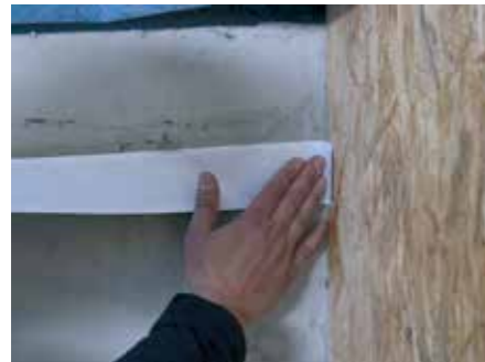
1. Position Tyvek® Butyl tape onto surface and press firmly into place
