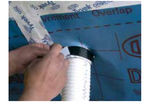
3. Remove the 2nd backing strip
