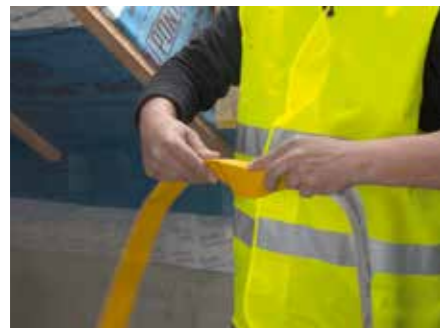
7. Fold Tyvek® Tape and remove smaller release liner strip
