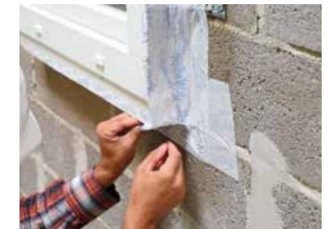
9. ...and dress around window frame, pressing firmly into place
