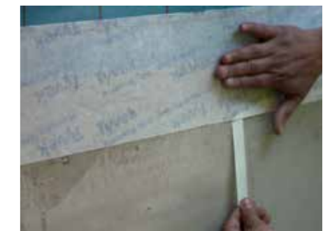
12. Remove remaining release liner and press tape firmly into place
