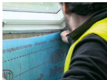
10. Position pre-cut AVCL and press against exposed tape adhesive applied earlier
