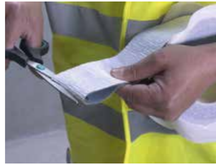
2. Cut off a small length of Tyvek® FlexWrap EZ
