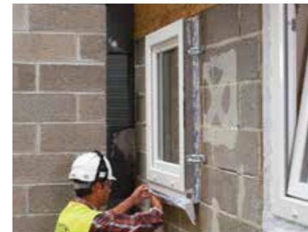
4. Fit the tape to the window cill first and press firmly into place
