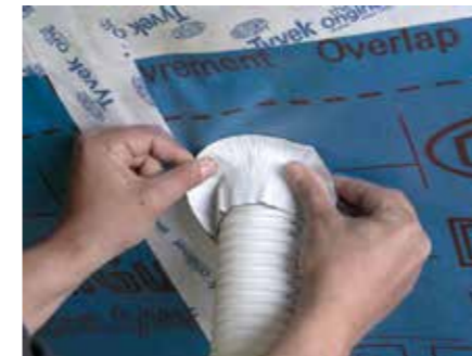
4. Fan the tape out onto the membrane, starting at the centre of the strip
