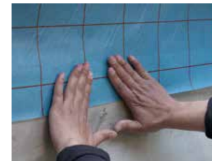
8. Fold DuPont™ AirGuard® AVCL onto primed surface
