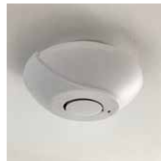
Mains smoke alarm
