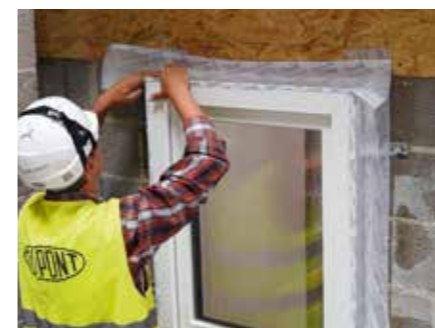
10. Complete the sealing work at the window head
