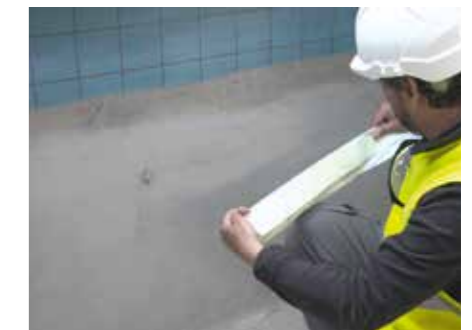
9. Prepare Tyvek® Window/Plastering Tape by folding back along the first split liner
