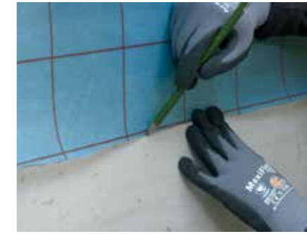
2. Mark out area where primer is to be applied
