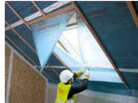
3. Cutting the vertical portion
