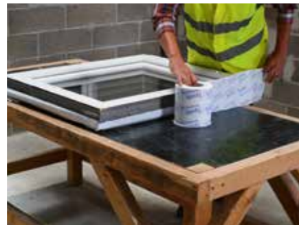
5. Turn the window over to prepare the inside
