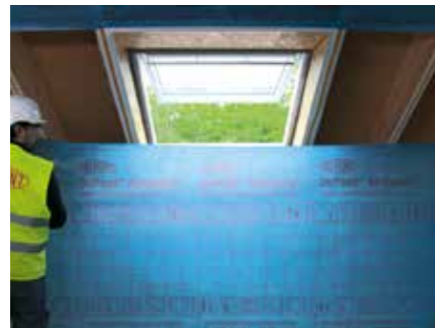
5. Measure required length of DuPont™ AirGuard® AVCL. Installation should start with the uppermost layer
