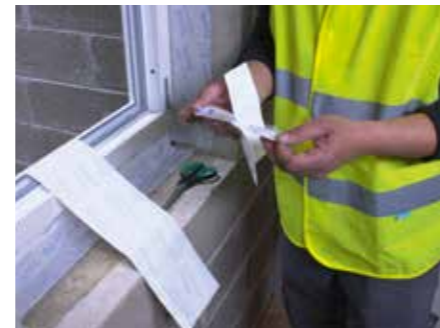
6. Remove a quarter of the release paper from the back of the tape
