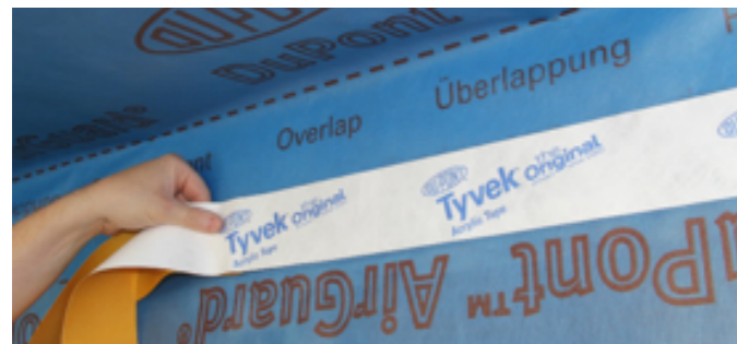
Maintain 100mm laps between each sheet and seal with Tyvek® Tape or Tyvek® Double-sided Tape (acrylic adhesive).
