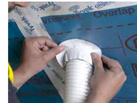
5. Press firmly to establish seal
