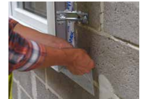
6. ... dress the tape around the detail and press into place
