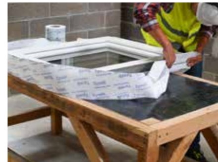
6. Repeat the same procedure as for the exterior side of the window. This time remove the large release liner of the tape (6 cm) and apply Tyvek® Window/Plastering Tape to the window frame
