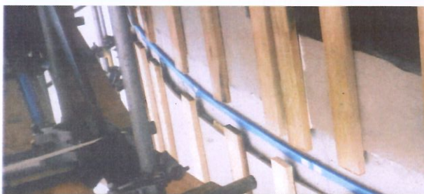
CV30 CAVITY BARRIER
