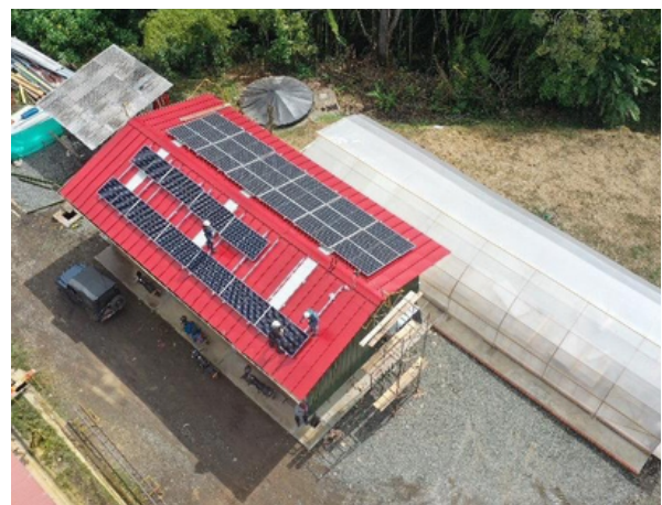
Solar Panels Installation
