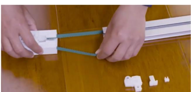
Make sure the wheel of the runner wheel goes in after the buckle the wheel must not go into the track ahead of the belt.
