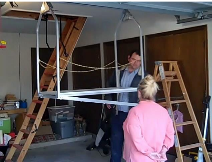
PHOTO SHOWING INSTALLER PULLING DOWN ON SPRING LOADED CEILING COVER. As the lift goes up through the opening, the cover catches on the ceiling allowing the springs to hold it tight. Lift shuts off automatically up and down.
