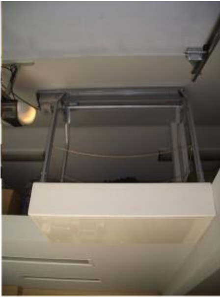
This Messinine install shows the ceiling Cover Underneath. (above)
