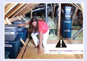
**Problem:** Entering or exiting the attic from a steep ladder is very dangerous without a hand-railing to hold onto and the unguarded ladder opening is a constant falling hazard while you are walking around and working in the attic!
