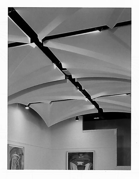
HYDROCAL FGR Gypsum Cement can be cast into lightweight, interior architectural elements, like these tent-shaped light coves, giving you the freedom to change the atmosphere of a space without expensive reinforcement costs.
