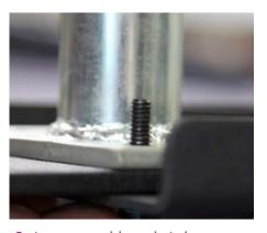
Insert and hand tighten a hex bolt with a flat washer from the bottom of the plate, so that the end of the bolt is exposed on top. Repeat for the other side.
