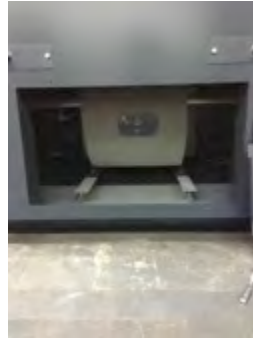
2. Remove access door to blower. See above pictures for location and access to recirculation blower.
