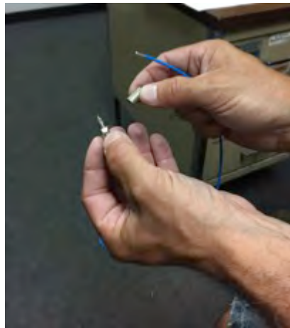
4. Inspect flame rod wire. If it is brittle and cracked, replace it. See fitting connection instructions on page 2.
