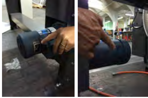
Belt motor brushes for excessive wear. Replace if necessary
