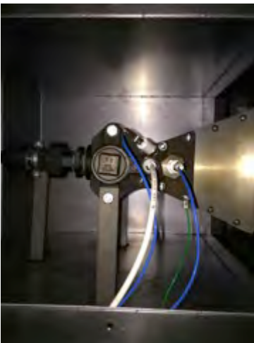
3. Inspect flame rods and wiring (blue wire). Clean flame rods using fine sand paper. If the rods are pitted and chipped, replace them.
