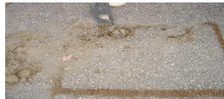
**Step 3:** Using a 24 inch level, check the bottom of the hole surface for level, and then place the pattern in the hole to check for size.
