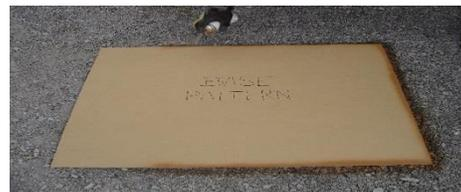
**Step 2:** Remove ground material from marked area until hole is approximately 3 inches deep. (As an option, you can remove 4 inches of material and add 1 inch of sand for ease of leveling.)
