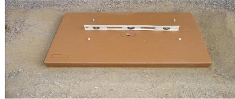
**Step 5:** Using a mini sledge hammer, pound the stem anchor into the ground or optional wet concrete through the hole in the center of the base. Make sure the top of the stem anchor is below the surface of the base.
