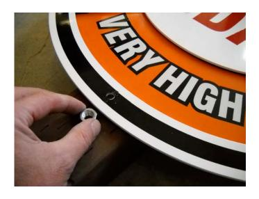
Use a 7/16" nut spacer/stand-off between the post and the back side of the outer sign at both the top and bottom holes. Attach sign to post using 5/16" x 2 ½" lag screw with flat washer.
