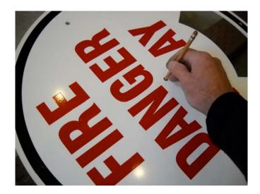
Place the sign on the post, a minimum of one inch from the top of the post. Mark the three mounting holes.
