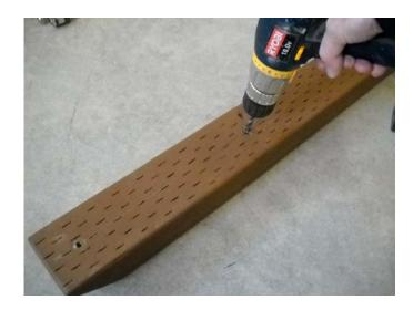
Pre-drill the three mounting holes using a 1/4" drill bit.
