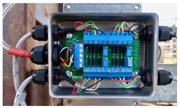
Connect the Digital Weigh Indicator cable to the <u>center</u> slot on left provided (as above) Connect load cell cables in this colour order: Black, White, Yellow, Green Red
