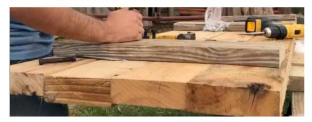
**Step 2** : Turn the platform upside down and use the spacers provided to drill  $2 \times 10^{12}$  holes at each corner of the platform. Space these holes and the load cells close to the edge of the platform.
