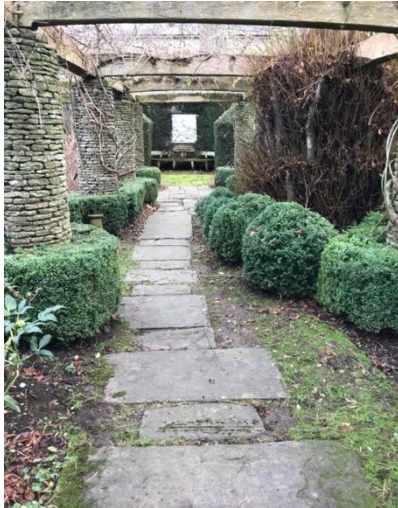
Irregular paving in the Pergola
