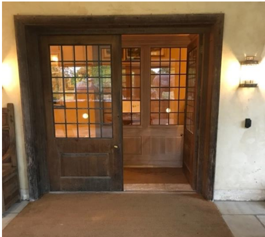
Doors into the Orchard Room
