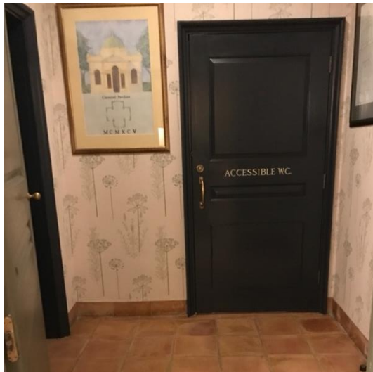
Accessible toilet outside
