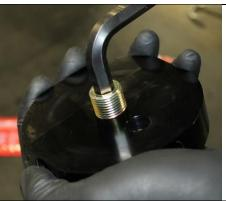
Before placing the filter head on the bracket. Assemble the straight NPT and ball valve and thread into the "IN" port, using sealant or pipe tape on threads.
