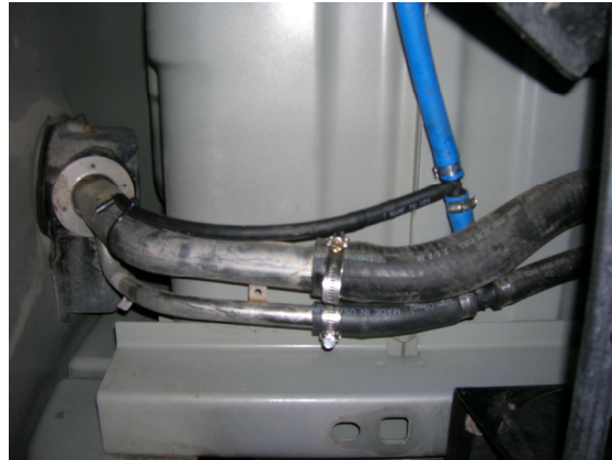
(Fig. 8) Photo shows final installation of fill hose and vent line hoses on vehicle's fill spout. Note the 1/4" Vent Kit Assembly hose is securely fastened to the fill spout. The 1/4" vent is necessary to prevent vacuum build-up in your TITAN™ fuel tank.
