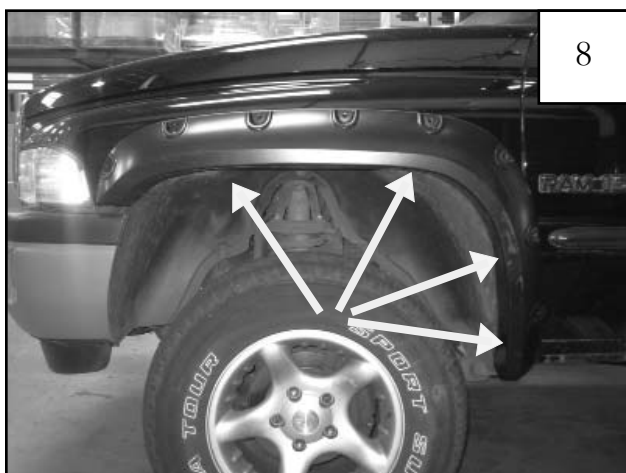
Using a right-angle drill with a #2 Phillips bit, drill four supplied Screws (SW1-0066) through plastic of fender flare and into sheet metal of fender using the indents in the flare as a guide. Install Screws from front to back.
