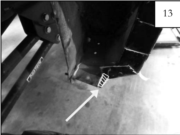
Using a Sawsall, cut off outlined area.
