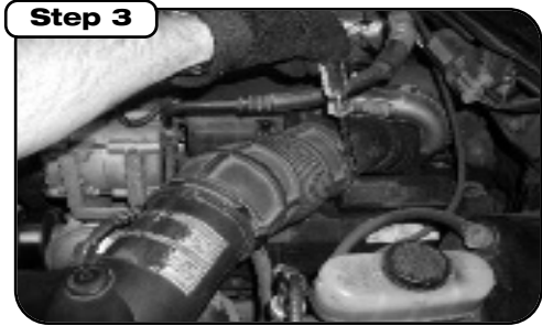
Loosen clamps securing stock intake tube onto stock air box and turbo inlet elbow
