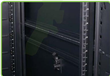
The vertical rails can be adjusted in quarter-inch (6.4mm) increments covering any mounting requirements for IT equipment. U positions are numbered for rapid installation of equipment.
