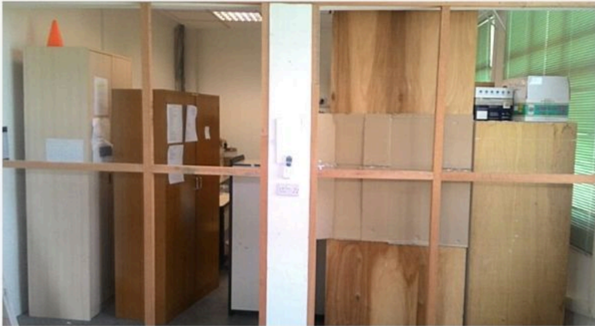
1st - nailed the plywood
