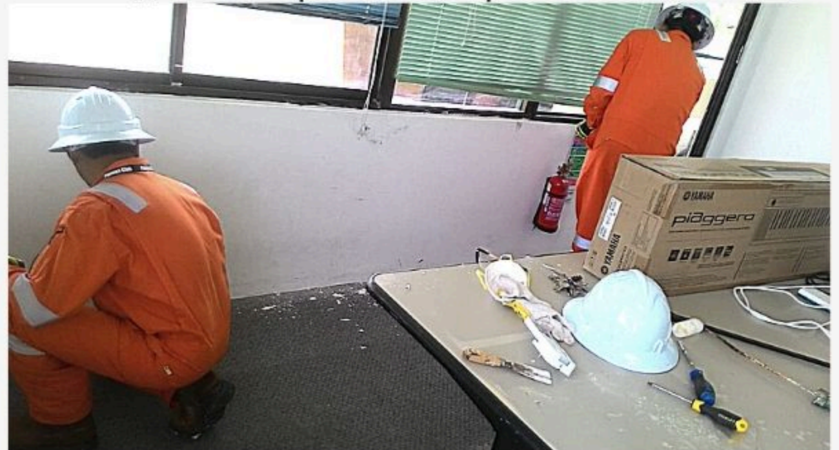
4th - scraped and repainted the room
