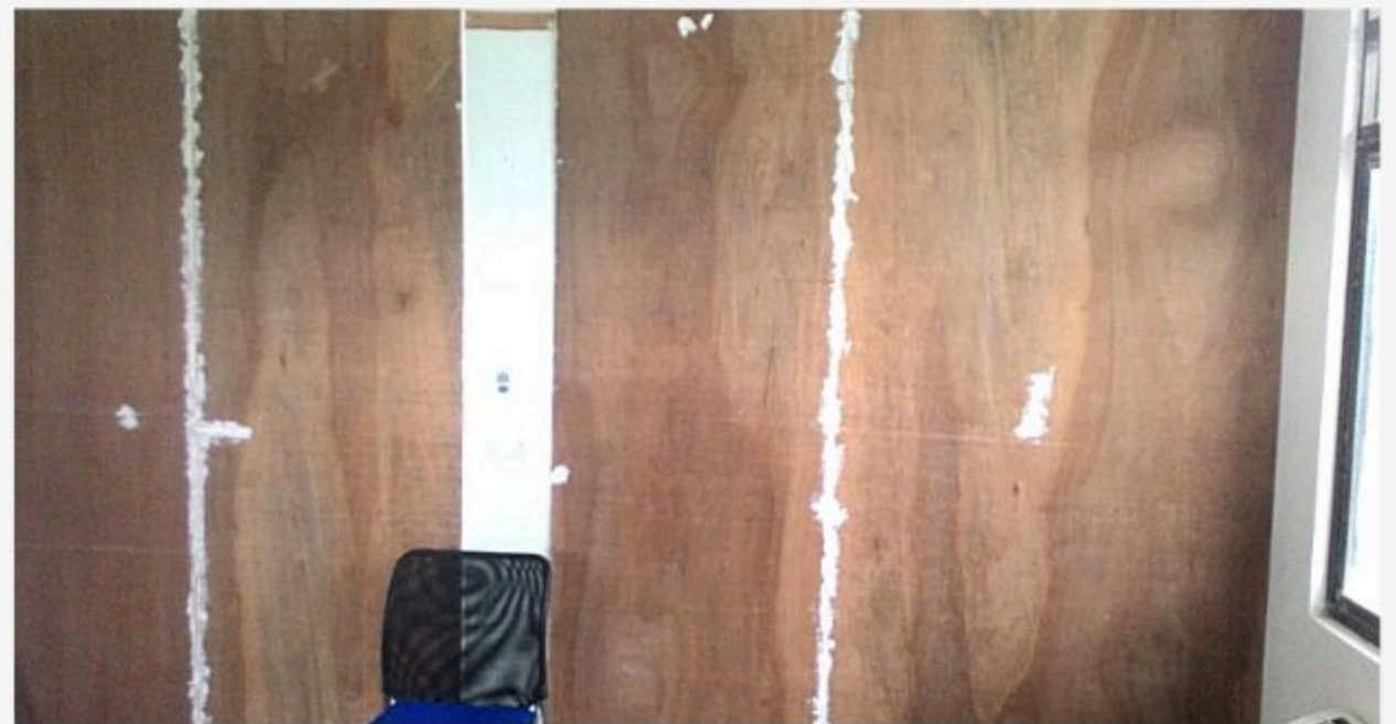
2nd - plastered the walls
