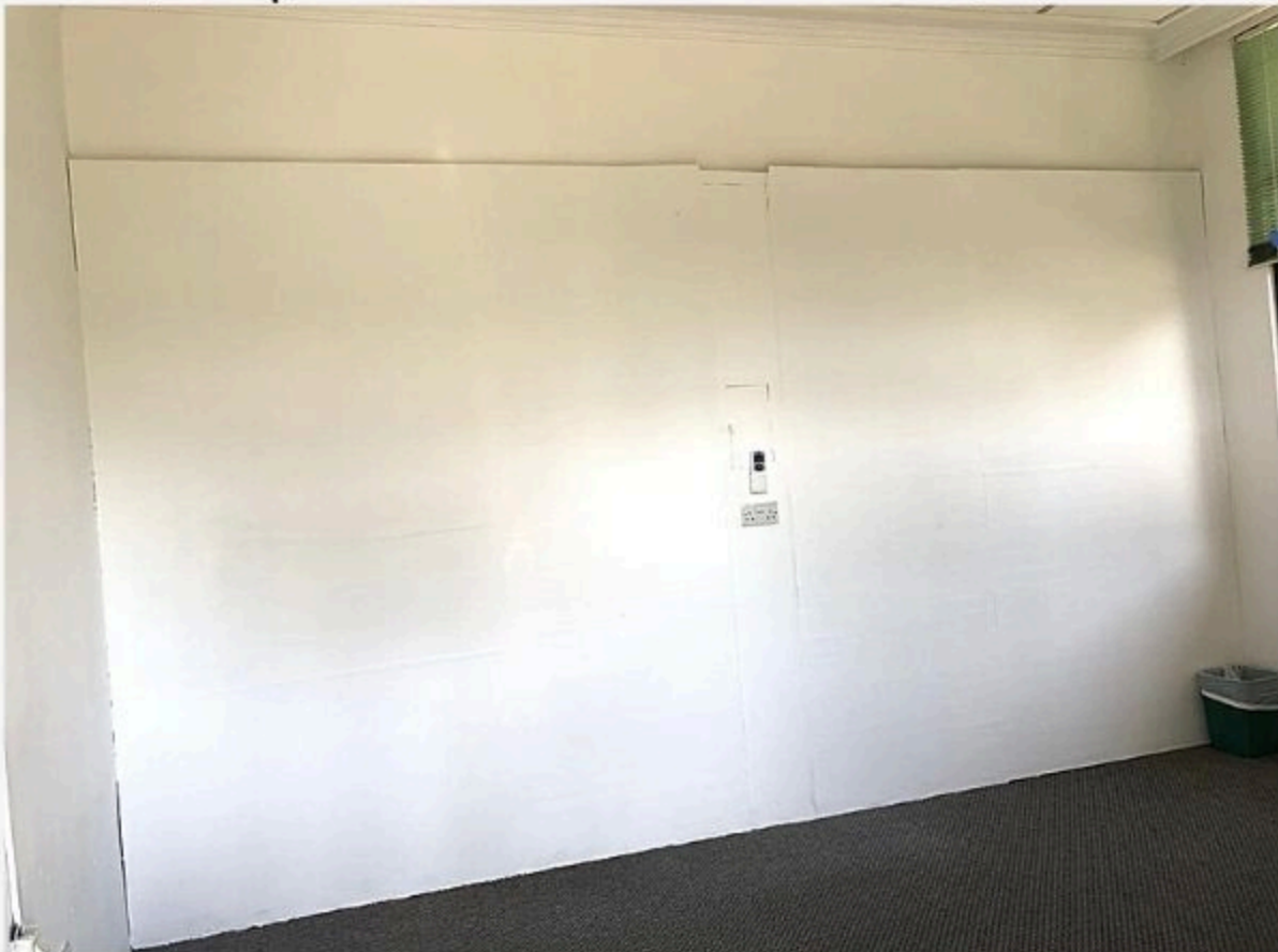
3rd - painted the wooden walls
