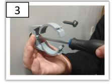
Use1/4" Wood Screw for Wood Installation.
