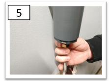
Route Cold Water Supply Line to Bottom of Unit and secure with Wrench.
