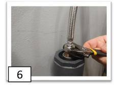
Attach provided ½" Supply Line from Unit to Faucet and SECURE with Wrench.
