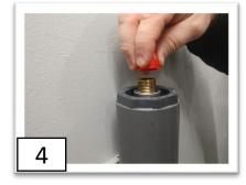
Cut Side of Cap and Remove Thread Protector.
