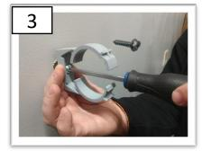
Use1/4" Wood Screw for Wood Installation.
