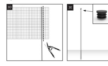
**3D.** After the upper wire mesh is secured fully to the span including both corners, cut away any excess wire mesh fence.
