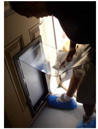
Clean the pet door frame and flaps thoroughly to remove any dust or fingerprints.
