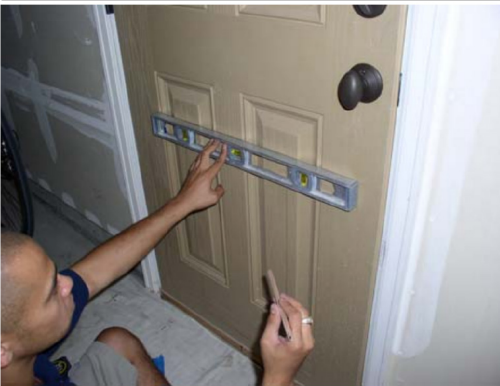
Make sure the opening is square and level before drilling. This will help ensure that the pet door operates correctly.
