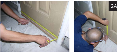
Measure and mark all four sides before making any cuts. Use a pencil or even masking tape to mark the square.
