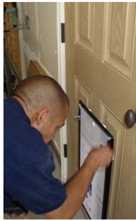
Clean the pet door frame and flaps thoroughly to remove any dust or fingerprints.
