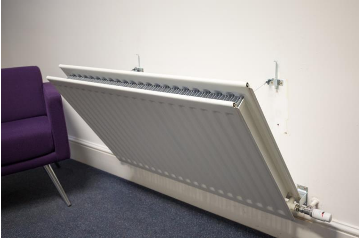
Figure 1. Example of Rotarad bracket and mount system which allows radiator to swing away from wall for cleaning and decorating access.
