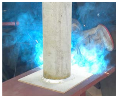
Fig.11 Field Welded Base Plate
